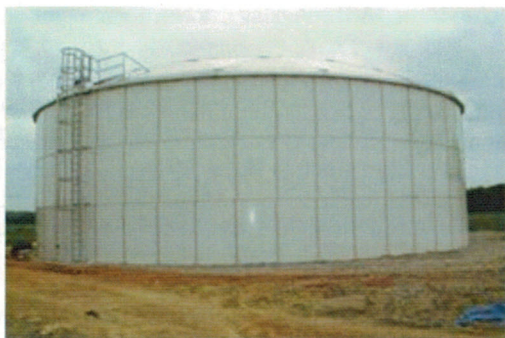
Figure 4: Fire protection water storage tank.
